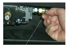
Adjustment Wire - Pull down to open or push up to close aeration cap.
